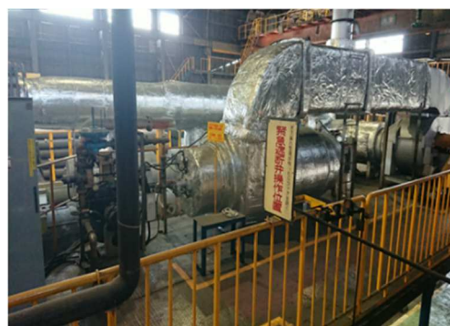
Toyama Plant: Thermal insulation work for the impregnation drying oven
