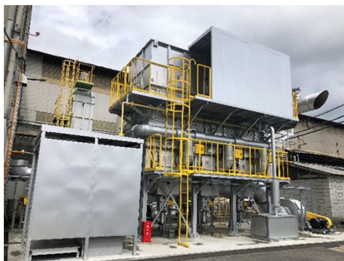
Replacement of the exhaust gas treatment equipment
